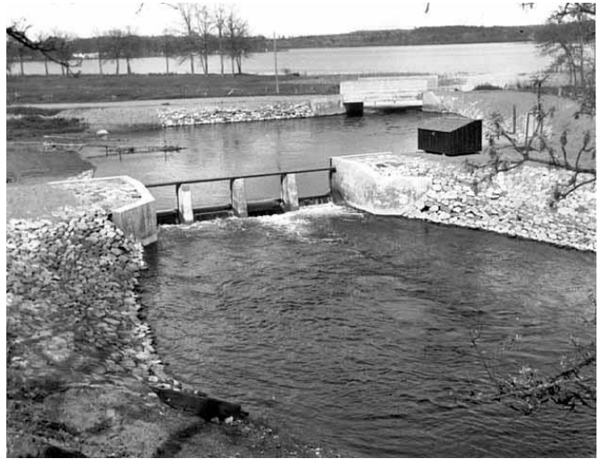
Lower South Long Lake Dam - completed 5/22/1937
